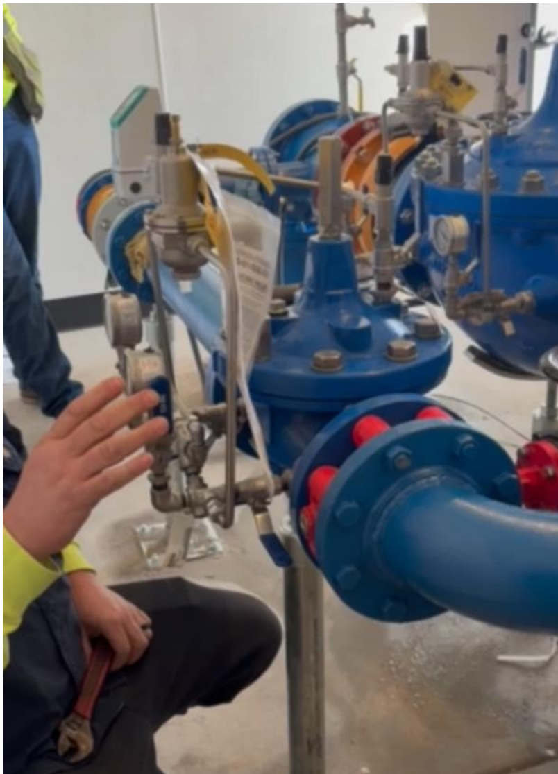
Final Startup of the Control Valves, part of Browns Canyon Connection
